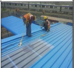
Uses of Life lines and mobile grab fall arrester for roof sheeting work.
