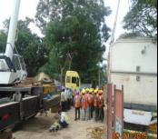
MS/RA on Lifting Of Machineries briefed and Pooja done before lowering of Flash Butt Welding Machine at Egmore tunnel & M/C was safely lowered on 09.01.2015
