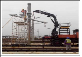
Two track cantilever erection using Unimog and trolley
